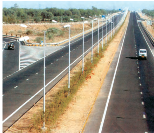
Fig. 7.2: Ahmedabad- Vadodara Expressway
