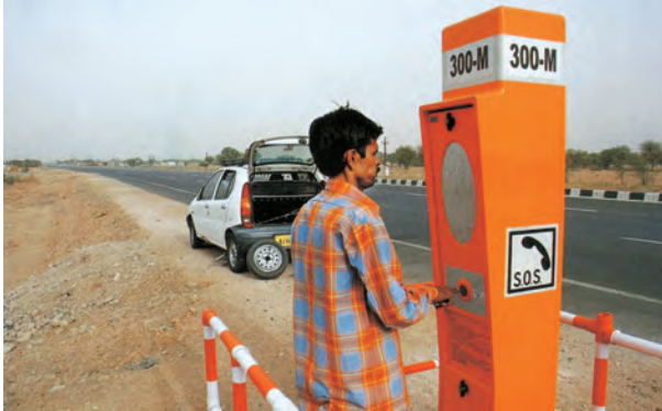
Fig. 7.10 : Emergency call box on NH-48
